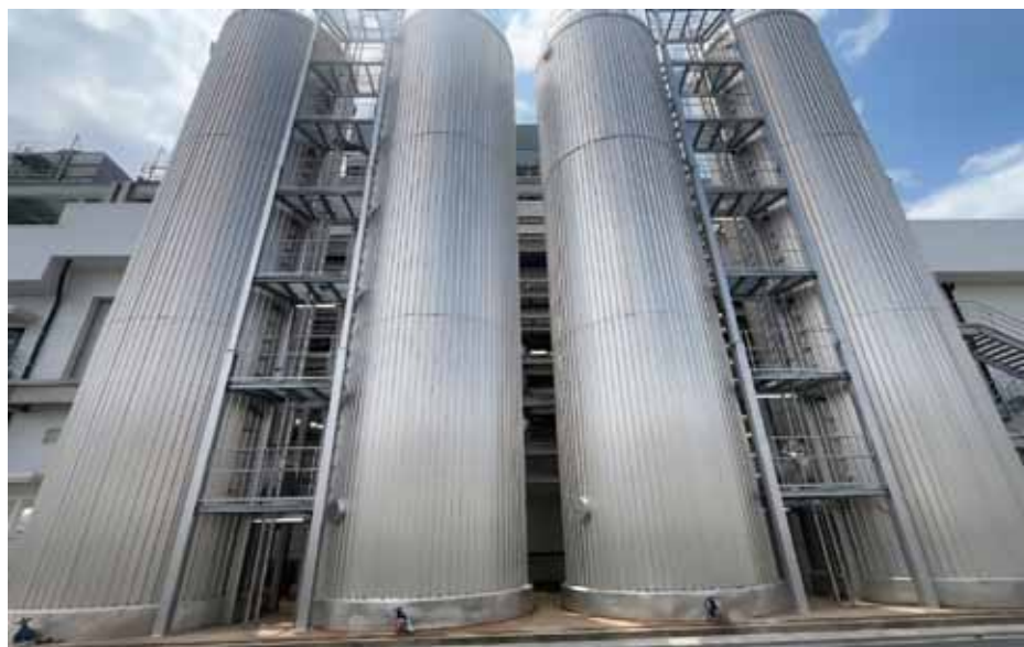
Largest buffer tanks in Malaysia (300m 3 ) built by LF Lansen
